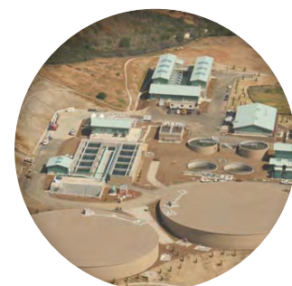
Twin Oaks Valley Water Treatment Plant
